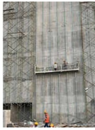
Construction Suspended Working
