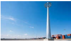
High Mast Pole
