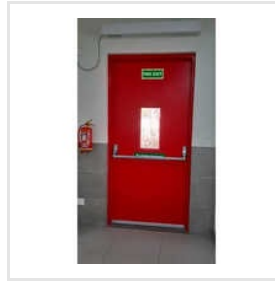
Emergency Fire Exit Single Door
