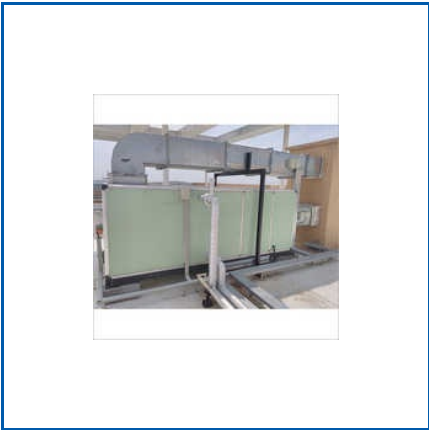
AIR HANDLING UNIT
