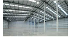
Prefabricated Factory Shed Fabrication
