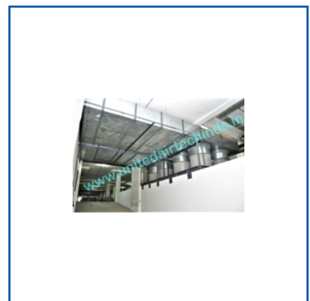
INDUSTRIAL DUCTING SPLIT PIECE SS DUCTING WITH AIR VENTILATION GRILLS PAINT BOOTH EXHAUST SYSTEM
