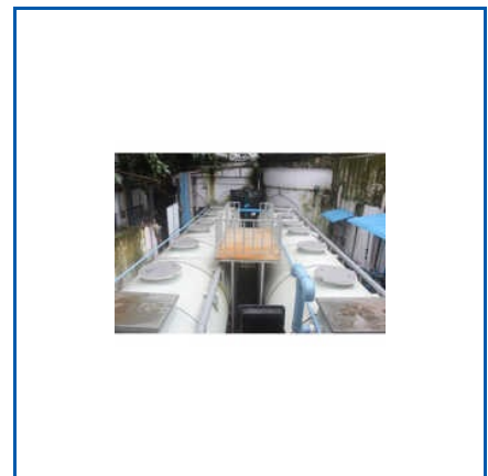
PACKAGED SEWAGE TREATMENT PLANT
