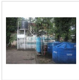
Sewage Treatment Plant
