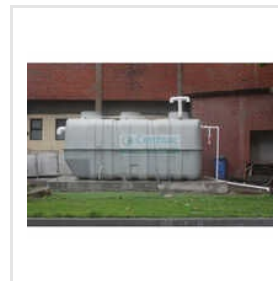
15 Sewage Treatment Plant
