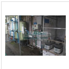
Sewage Treatment Plant At Mumbai
