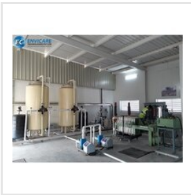
Civil Sewage Treatment Plant
