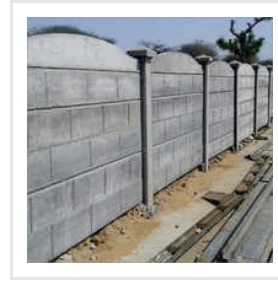
RCC Boundary Wall
