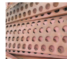
GD Screen at Inlet & Outlet
