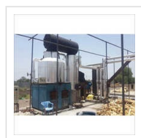
Solid Fuel Fired Thermic Fluid Heaters
