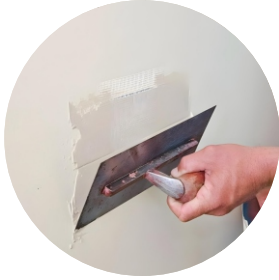
Plaster Repairs
