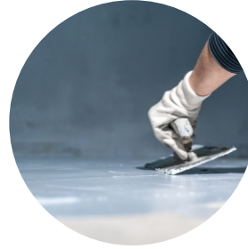
Bathroom Waterproofing
