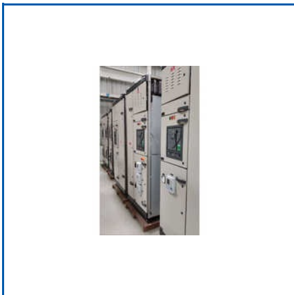
PCC CONTROL PANEL
