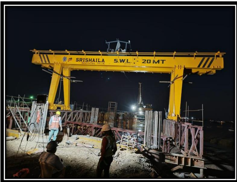
Double Girder Gantry cranes are more suitable for carrying heavy & critical load for longer bay length and heavy duty operations.
