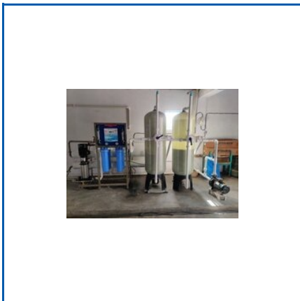
4000 LPH INDUSTRIAL RO PLANT
