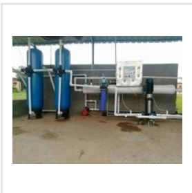
4000 LPH Mineral Water Plant
