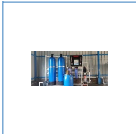
DRINKINGI WATER PLANT
