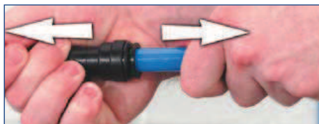
3. Pull on pipe to check secure.
