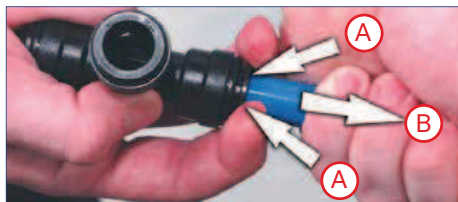
3. Pull on pipe to check secure.
