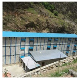
G2 Workers Accommodation
