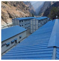
Prefabricated Labor Colony
