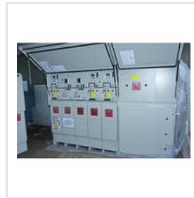
11 KV Siemens 5 Way Ring Main Unit
