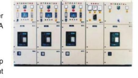
Bus bars designed for upto 4000A at 50kA (rms) for 1 Sec, fault Level
