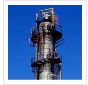
Distillation Column And Pressure Vessels
