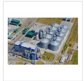
Commercial Modular Refining Plant
