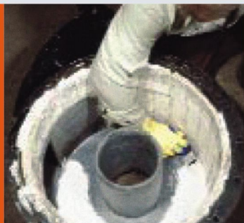
Inner Base of Dust Collector Coated with Aluma-Coat TW
