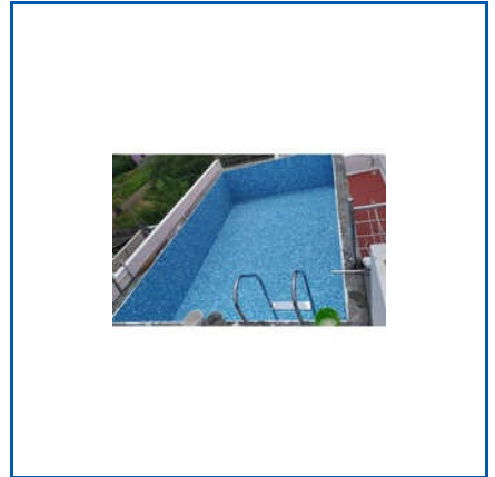
SWIMMING POOL MAINTENANCE SERVICES
