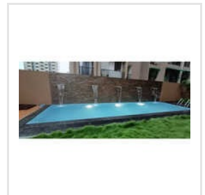
Swimming Pool Renovation Service
