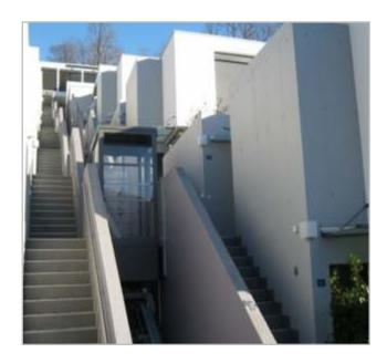
An Incline Elevator is an elevator that runs in a direction diagonal to the ground. Unlike a standard elevator, incline elevators can go up tilted grades.
