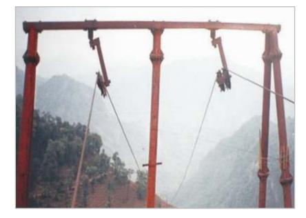
A Mono-cable system has only one cable that does the work of supporting and also propelling. The carriers may also be detached from the cable.
