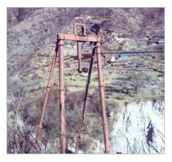
A Bi-cable system has two cables, one of which supports the carriage (track rope). This cable is stationary while the other cable (hauling rope) moves and serves the purpose of propulsion.
