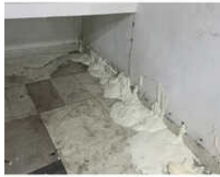
Polyurethane Injection Grouting Services
