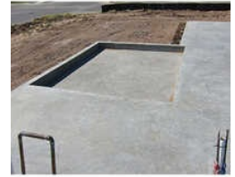
Bathroom Sunken Slab Waterproofing
