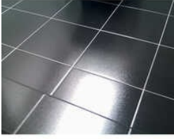
Tile Epoxy Grouting Services
