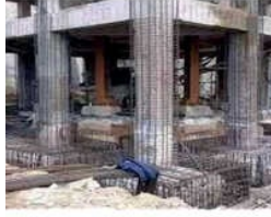
Structure Strengthening Services
