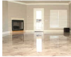
Epoxy And PU Flooring Services
