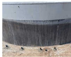
Cement Grouting Waterproofing
