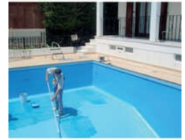
Swimming Pool Waterproofing
