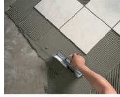
Tile Laying Services
