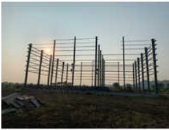
Pre Engineered Metal Building Structure
