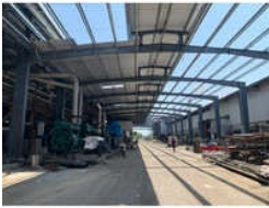
Industrial MS Pre Engineered Structure
