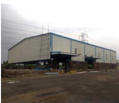
Pre Engineered Dal Mill Building
