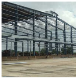
Pre Engineered Structure
