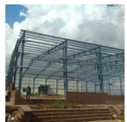
Pre Engineered Building Structure
