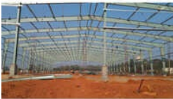
Pre Fabricated Structure
