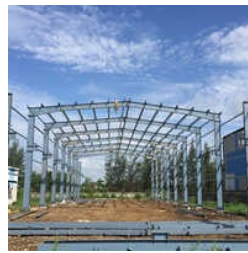
Steel Pre Engineered Building Structure
