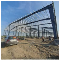
MS Prefabricated Building Structure
