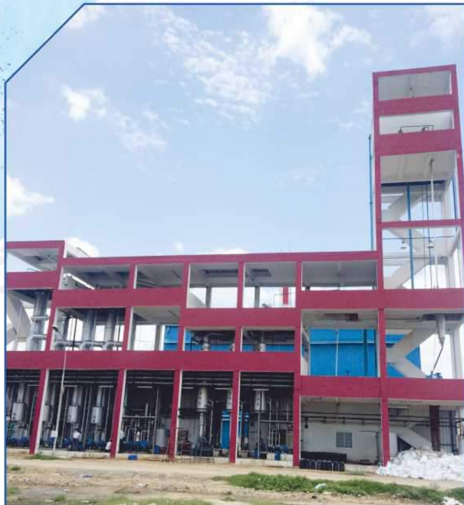
VANITEC CETP LTD 630 KLD
