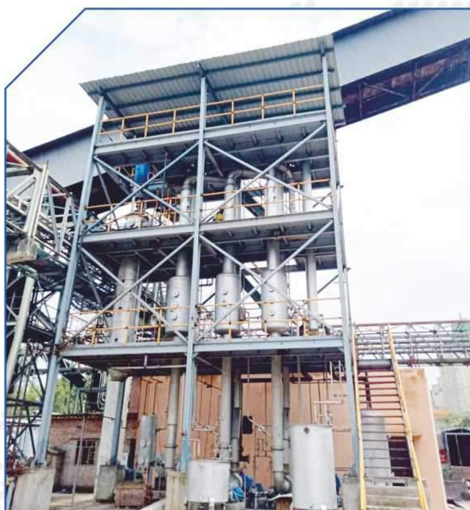
ACC CEMENT 60 KLD
