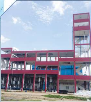
VANITEC CETP LTD 630 KLD
