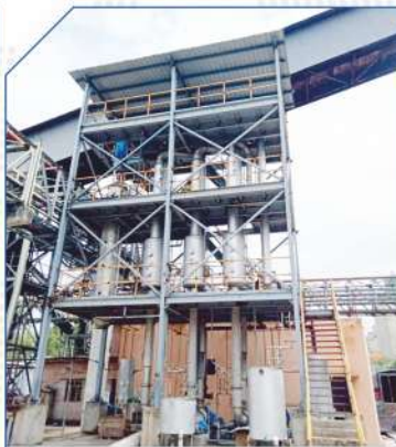
ACC CEMENT 60 KLD
