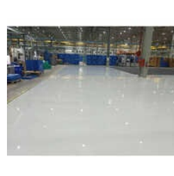
Self Leveling Epoxy Flooring
