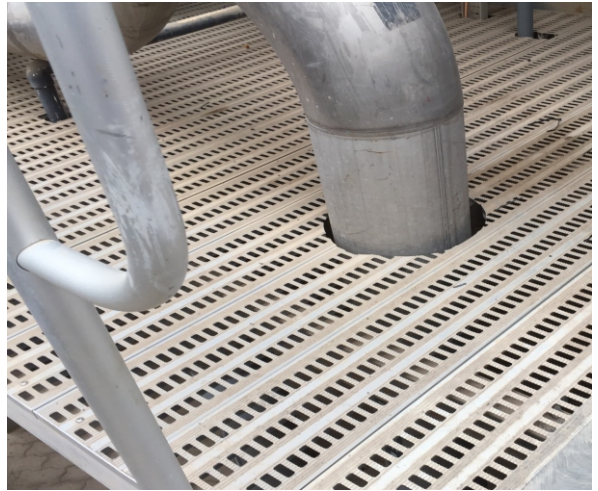
Installed Deck type Grating with cut out opening
