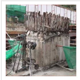
Diamond Wire Sawing Services
