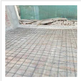
Chemical Rebaring Service
