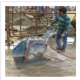
RCC Cutting Service
