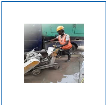
CONCRETE SLAB CUTTING SERVICE
