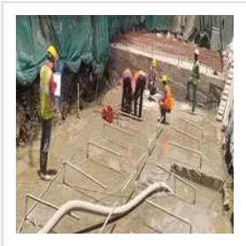
Floor Sawing Services
