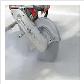
RCC Floor Cutting Services
