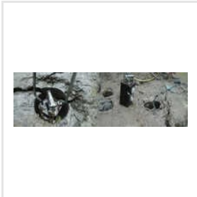
Concrete Hydraulic Splitting Service
