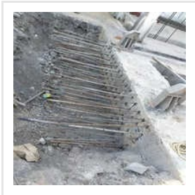
Rebar Grouting Services
