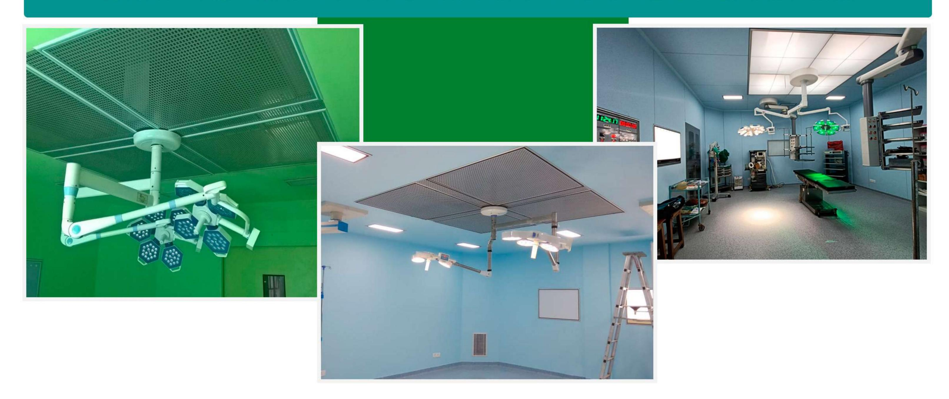
Ceiling Mounted Laminar Flow makes an integral application in Operation Theaters. Hospitals search for top quality Ceiling Mounted Laminar Flows to ensure ultra clean sterile HEPA filtered Class 100 first air into OTs where highly sensitive activities take place.
