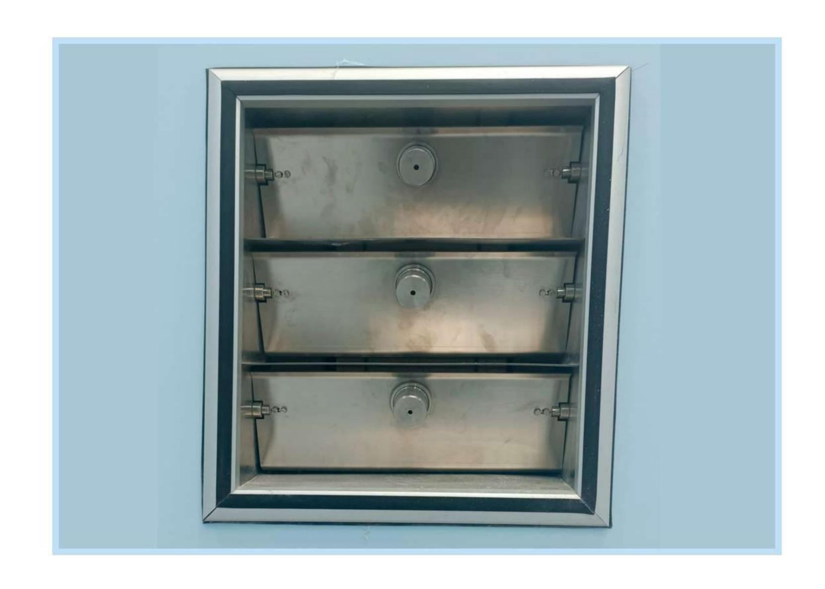
These dampers are back draft air damper that come along with the adjustable start-open pressure.
