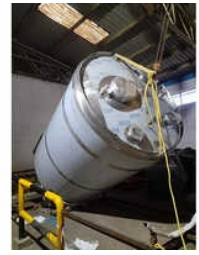
Stainless Steel Tank Installation Services
