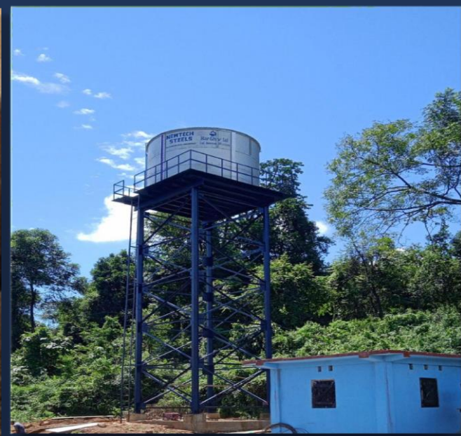
Self Elevated Tanks (on structure)
