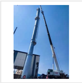
100 Tons Terex Crane Rental Service
