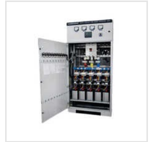
Capacitor Bank Apfc Panel
