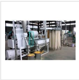
Semi Automatic Wheat Mill Plant Installation
