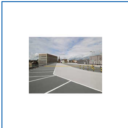
CAR DECK PARK FLOORING
