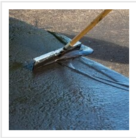
Coal Tar Coating
