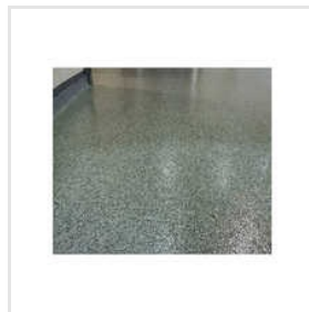
Granular Epoxy Flooring
