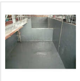
ETP Tank Coating
