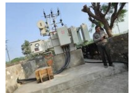
25 KVA Three Phase Distribution
