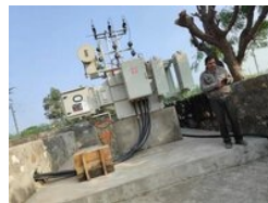
100 KVA Three Phase Distribution
