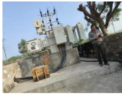
250 KVA Three Phase Distribution
