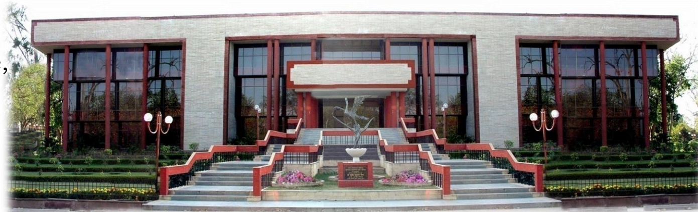
NCL Headquarters, Singrauli (M.P), designed and constructed in 2000 – 01
