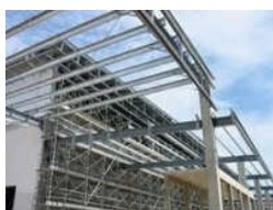
Industrial Structural Fabrication
