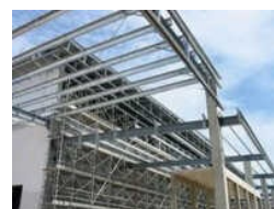
Metal Structure Fabrication
