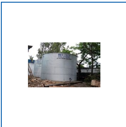
ZINCALUME RAW WATER STORAGE TANKS
