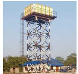
Amitex GRP Over Head Water Tank On Staging
