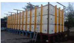
Amitex GRP Water Tank
