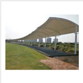
Car Parking Tensile Structure
