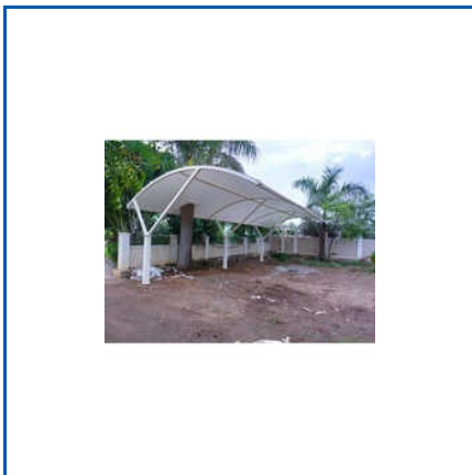
CAR PARKING ROOFING SHED
