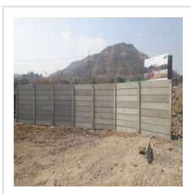
RCC Precast Security Boundary Wall
