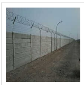
RCC Precast Boundary Wall
