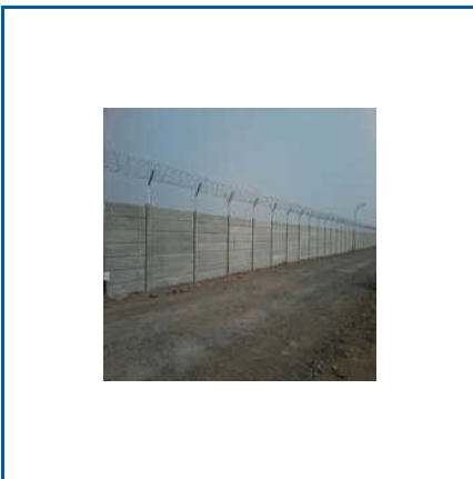
PRECAST BOUNDARY WALL
