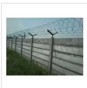
RCC Security Compound Wall
