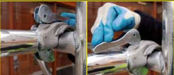
Cam-Lock unlocked
