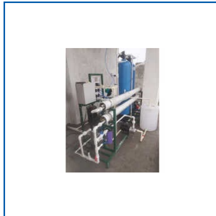
COMMERCIAL RO PLANT
