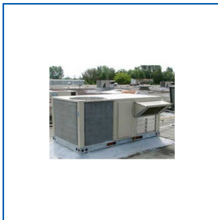
ROOF TOP AIR CONDITIONER
