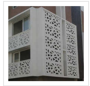
Cement Railing Jali
