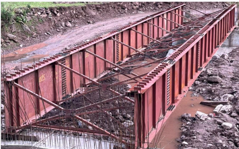
Plate Girder Bridge
