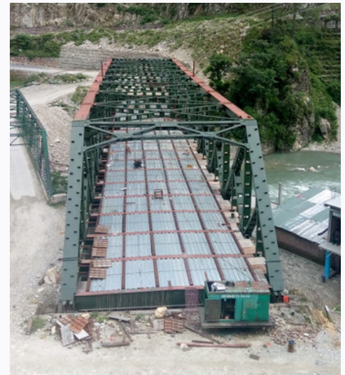
Steel Truss Bridge
