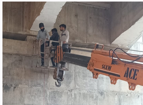
Old RCC Bridge Repaired by Epoxy Mortar & Injection Grouting
