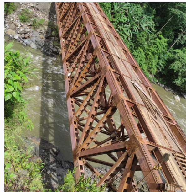
Deck Type Truss bridge
