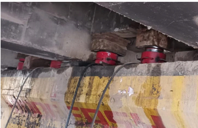
Lifting of RCC Bridge
