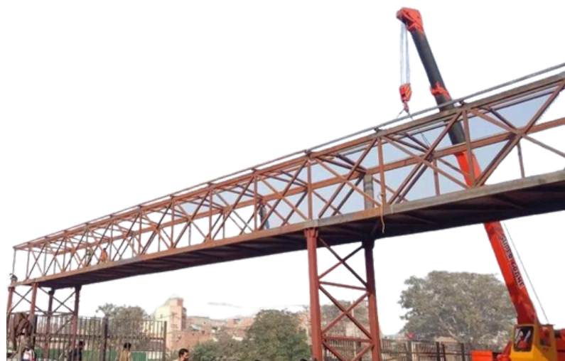
Foot over Bridge
