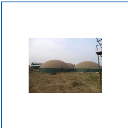
18000 M3 COMMERCIAL BIOGAS PLANT
